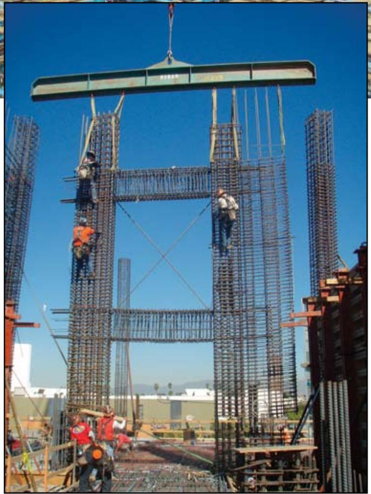
Shear wall rebar was detailed to allow pre-tying of cages offsite. This minimized field labor and accelerated construction.
