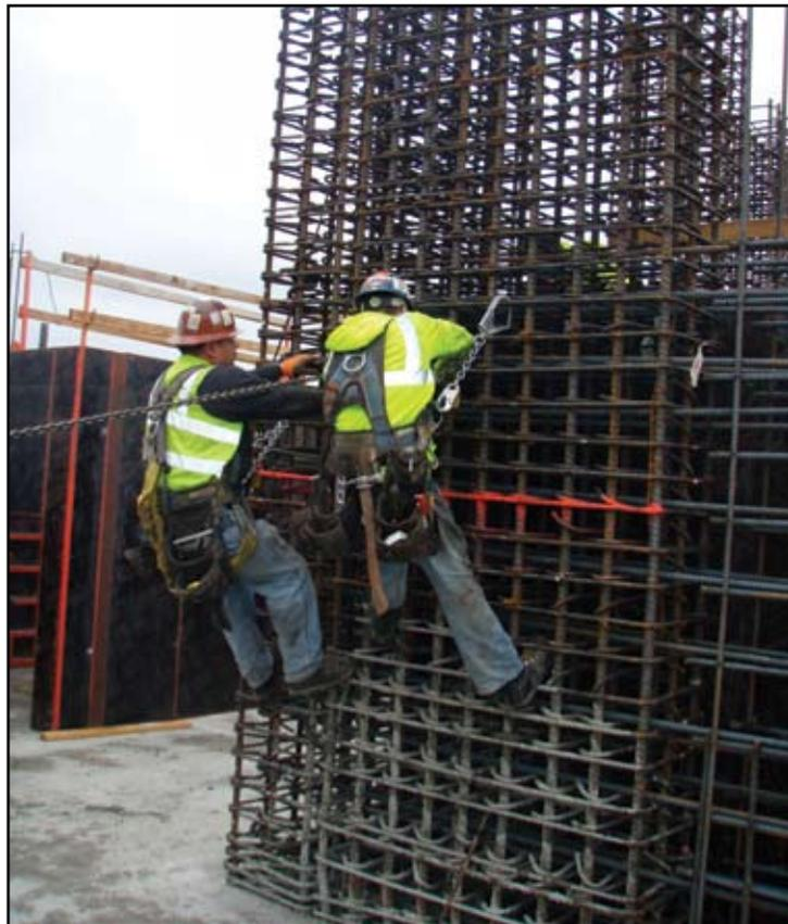
Rebar ties with a 90 ksi yield strength substantially reduced congestion at columns and shear wall boundaries.
