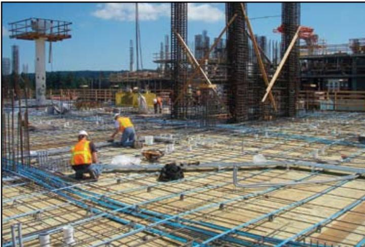
Slabs are typically 8-inch thick with a combination of post-tensioning and mild rebar. Note that exhaust ducts were buried in the slabs, along with most electrical conduit.
