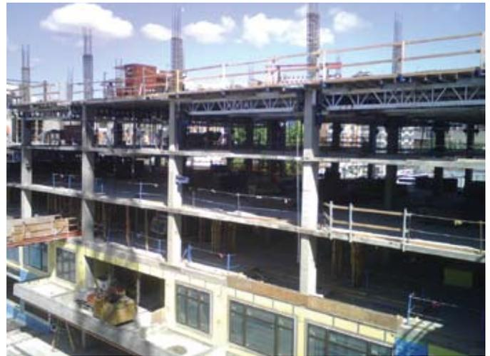
**Column-hung flying deck forms prior to placing the slab. All slab loads are carried directly by the columns, resulting in open decks below the forms with no shores or reshores. This allows workers to move about freely**
