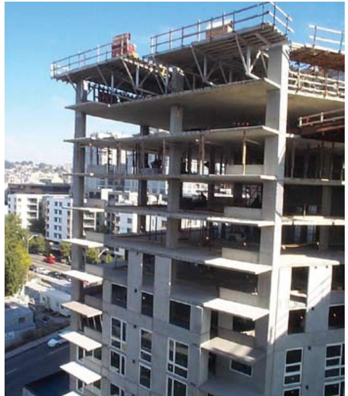
**Conventional flying form trusses immediately after flying. Reshores will be installed prior to placing the slab**
