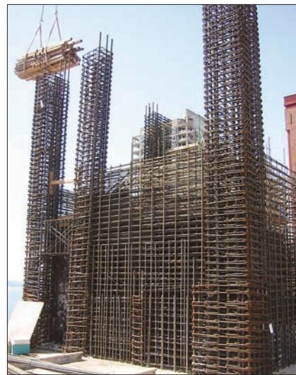
▲ Shear Wall. Boundary elements are simpler.
